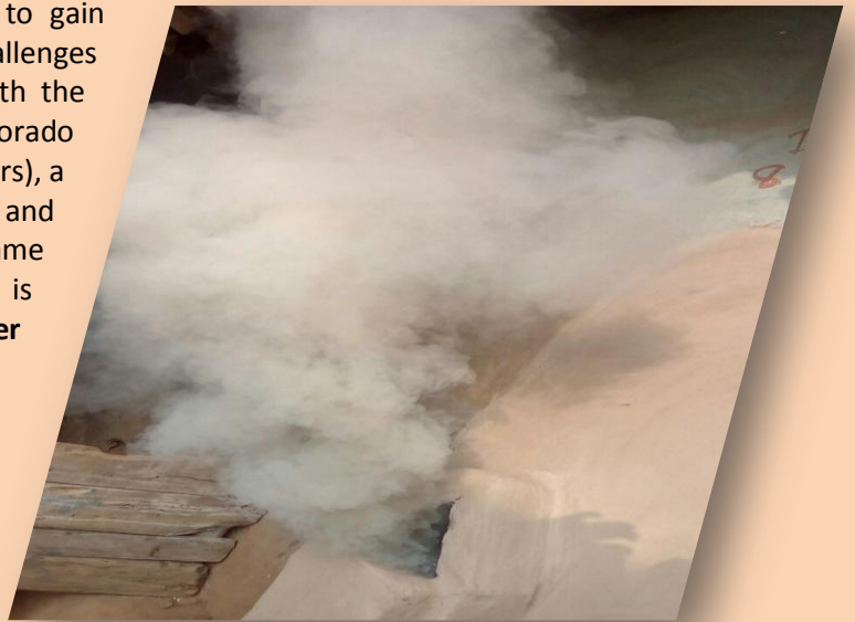
Smoke ventilating from the outlet outside the house.
