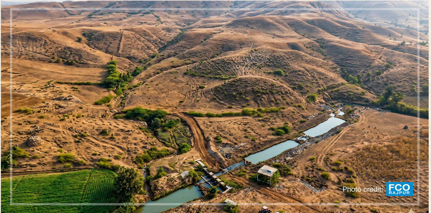
Small structures, big difference: A Doha in Temla village, Barwani district, Madhya Pradesh. Each structure lasts 5 to 7 years.
