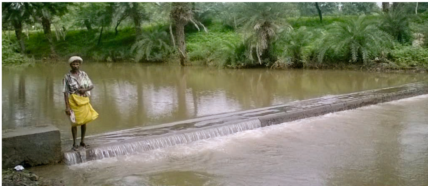
Anicut constructed in collaboration with PHE dept. under MGNREGS works providing technical support to Gram Panchayat Jhaua dist M.P.
